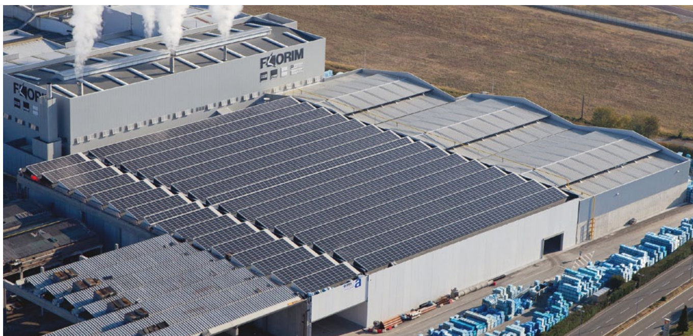
Solar panels – Factory in Fiorano Modenese (MO – Italy)
